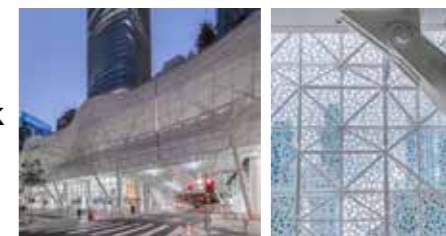
C Bus Deck Facade
