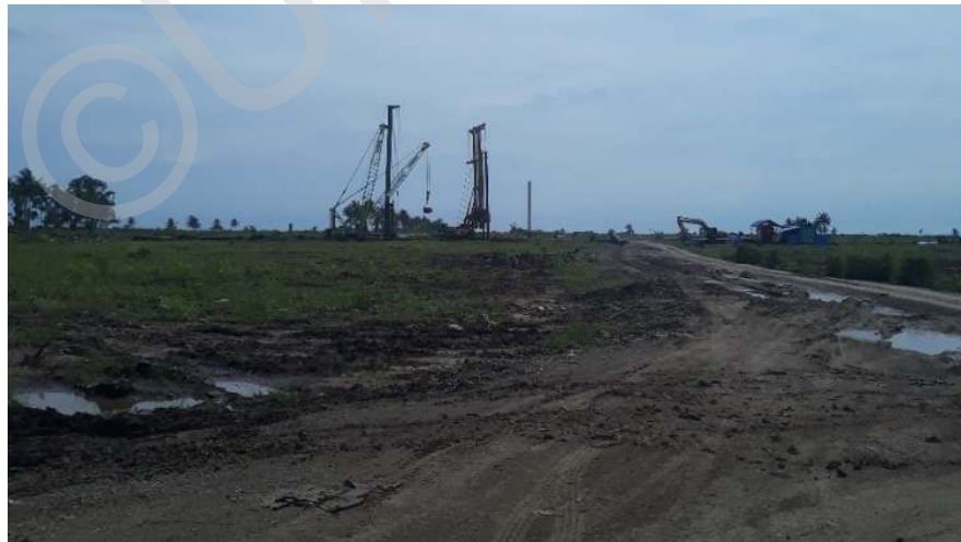
Gambar 02: Land clearing area lahan proyek Yogyakarta International Airport Sumber: Dokumentasi Mahendra, 2018
