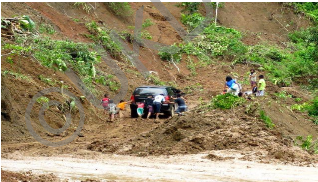
Figure 1.3: The road to Mamasa District. During this period, there were 136 potential landslides with the distance of approximately 80 km from the last paved road with traveling time up to 6 hours. Photo: Dhyana Paramita. 2016
