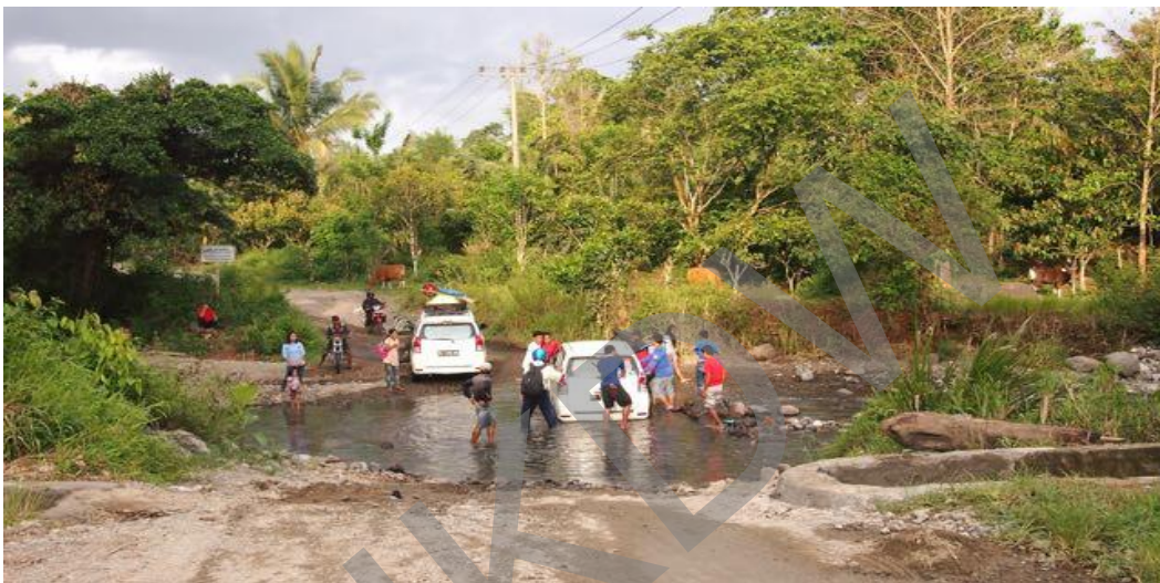
Figure 1.2 : The road to Bonehau Sub-District cut approximately by 25 big, medium and small rivers as well as massive pod-holes. During the rainy season the road could not be traveled. (Photo: Dhyana Paramita. 2016)
