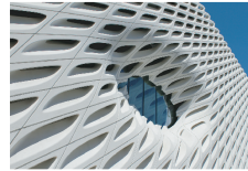
PELINGKUP LUAR BANGUNAN GLASS FIBER REINFORCED CONCRETE
